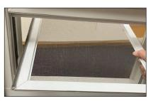
E. To replace, insert screen under the bottom sash and position the side with spring tension clips into screen rail enough to get screen to insert into opposite side screen rail. On
