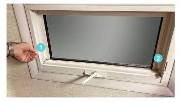
Then rotate the operator counter clockwise 3 until the sash is opened to the desired ventilating position.
