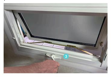
**To Close**: Rotate the operator clockwise until the sash gently contacts the awning frame. Then flip down both security locks to fully seal the operating sash.
