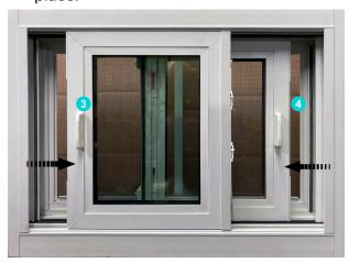
3) For a secure ventilation, unlock cam locks, pull vent latch out, 5 on outer most sash and slide inner sash until it stops at the steel spring ventilation lock, 6.
