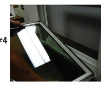
2. Grasp sides, swing sash up to about a  $45^{\circ}$  angle, # 4, to disengage it from locking shoe, tilt sash sideways and lift out. This will disengage the other side as well.
