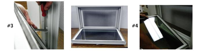
2. Grasp sides, swing sash up to about a 45<sup>o</sup> angle, # 4, to disengage it from locking shoe, tilt sash sideways and lift out. This will disengage the other side as well.
