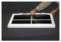
**3.** Grip the glazing bead in the center and remove it from the sash. Repeat the the same procedure (#2) to remove the remaining glazing beads.
