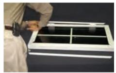
**6.** Repeat same actions as in (#5) on opposite side of sash. Remember to replace the short glazing beads first.
