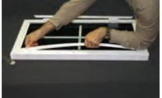
$m{7}ullet$  Replace the longer glazing bead sections in the same manner as (#5 and #6). After inserting corners and gently pushing bead into place, use a block of wood or the heal of your hand to snap the glazing bead into place.
