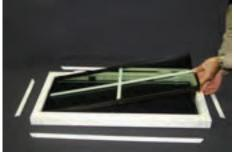
Now remove the glass and replace with new unit. If necessary, new adhesive backed setting blocks, that adhere to the sash frame, can be used to replace those installed during manufacturing.
