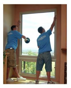
Recommended tapered shims should be approximately 2" wide. Place two shims at each shimming point, one from the inside and one from the outside for level support across the entire 3-1/4" depth of the frame.
